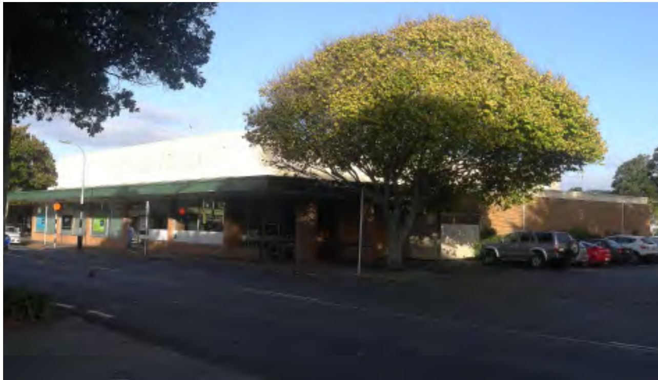
Former New World site. Planned for redevelopment for apartments.
