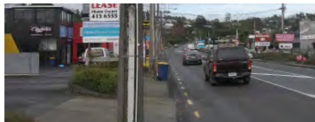
Beach Road has very low visual quality and in places presents a physically difficult environment for pedestrians.
